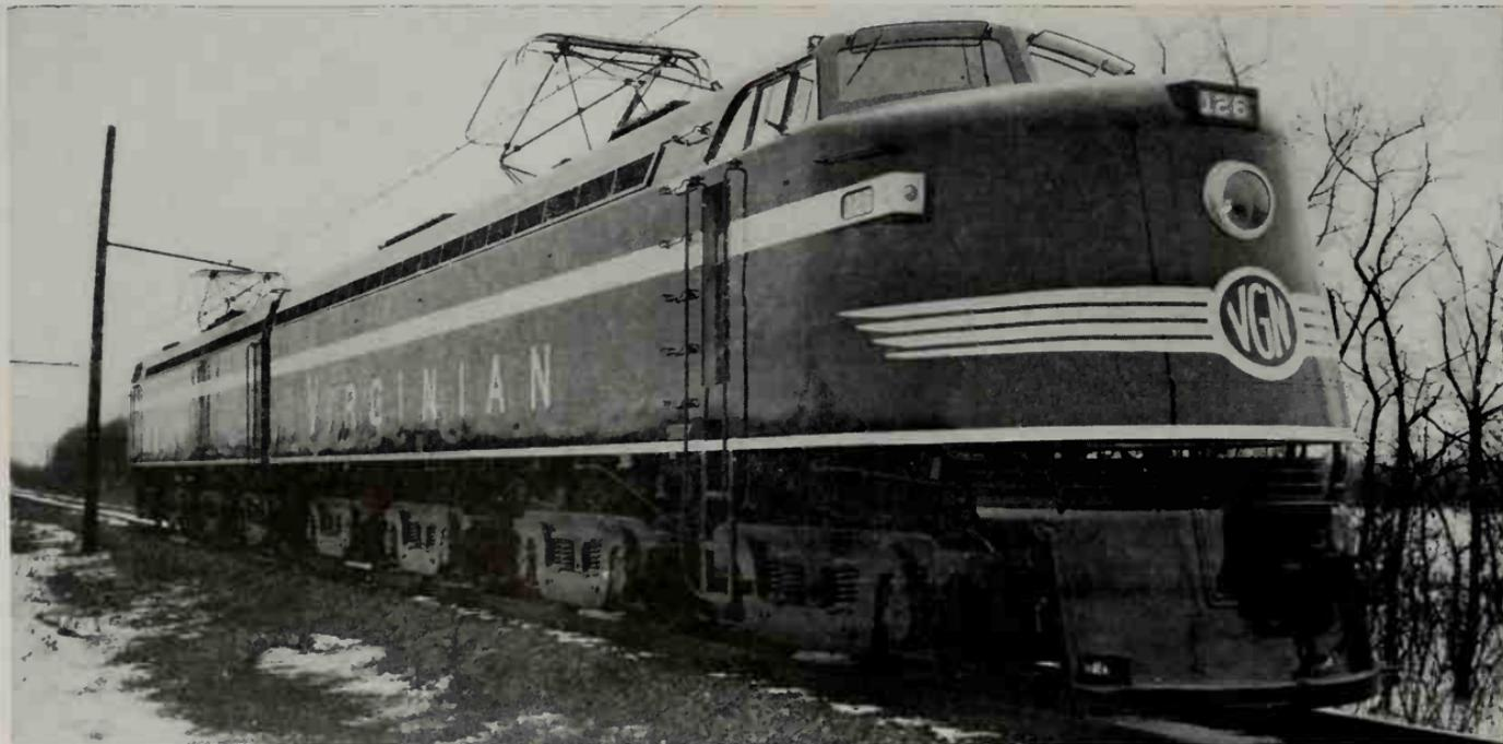
Virginian 6,800-hp. Motor-Generator Locomotive built by the General Electric Co. in 1948.
