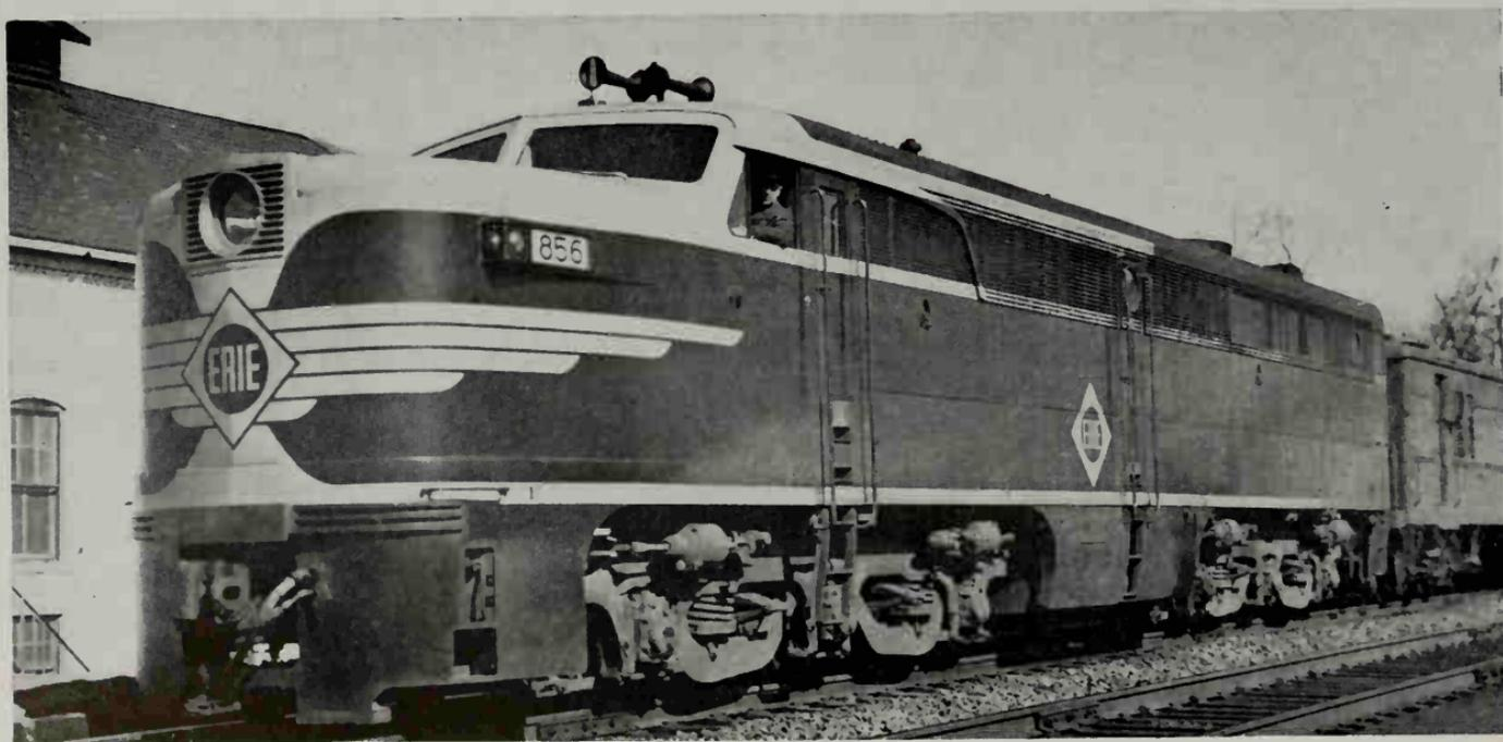
Erie No. 856, Class PA-20; 2,000-Hp. Passenger Locomotive built by American Locomotive Company-General Electric Company in 1949.
