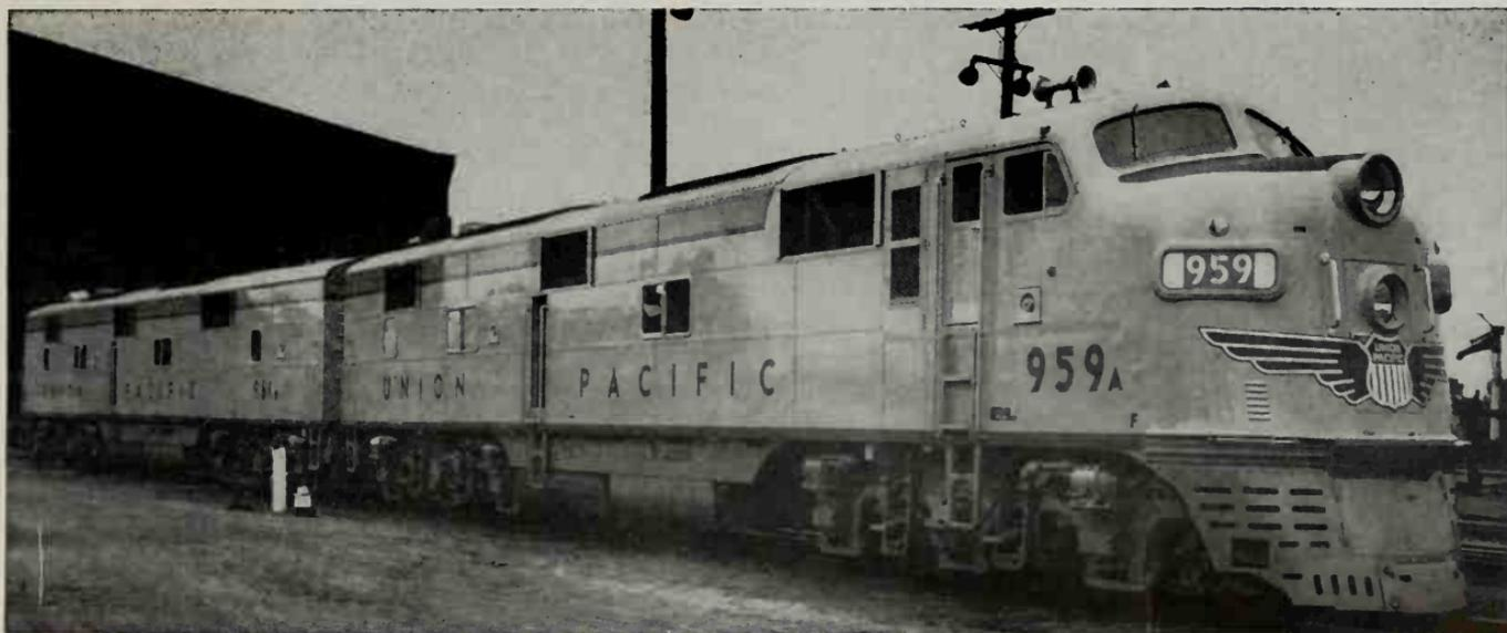
Union Pacific Nos. 959A & 961B, Two Unit 4,000-hp. Passenger Locomotive built by Electro-Motive Division—General Motors Corp. in 1946, Model E-7.
