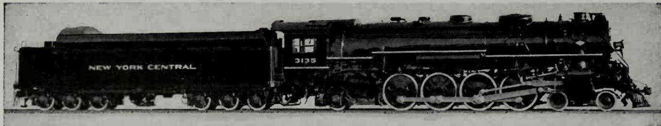
New York Central 4-8-2 (Mohawk) Type Locomotive for freight and passenger service, Class L-4a, Nos. 3100-3124 and Class L-4b, Road Nos. 3125-3149. Built by Lima Locomotive Works, Inc., in 1943.
