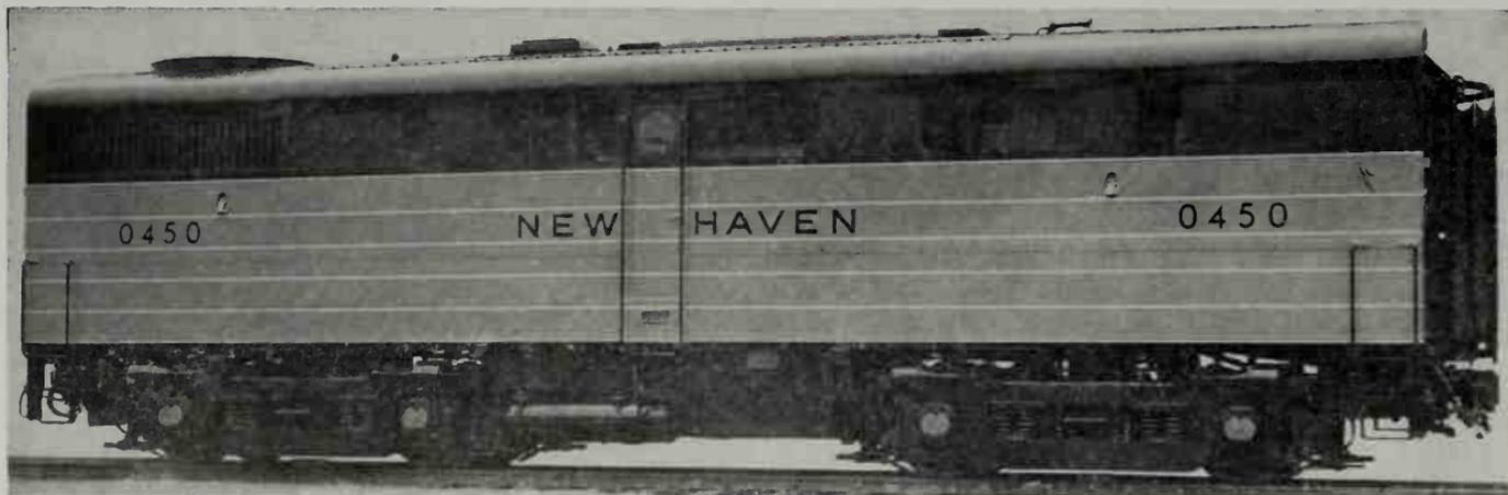
New York, New Haven and Hartford No. 0450; 1,500-Hp. Diesel-Electric Freight Locomotive, B Unit built by Alco-G.E. in May 1947.
