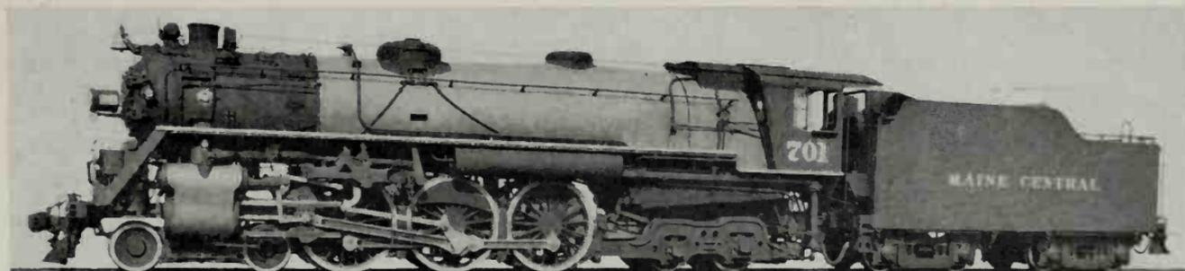
Maine Central 4-6-4 Type Locomotive for passenger service, Nos. 701-702. Built by The Baldwin Locomotive Works in 1930.
