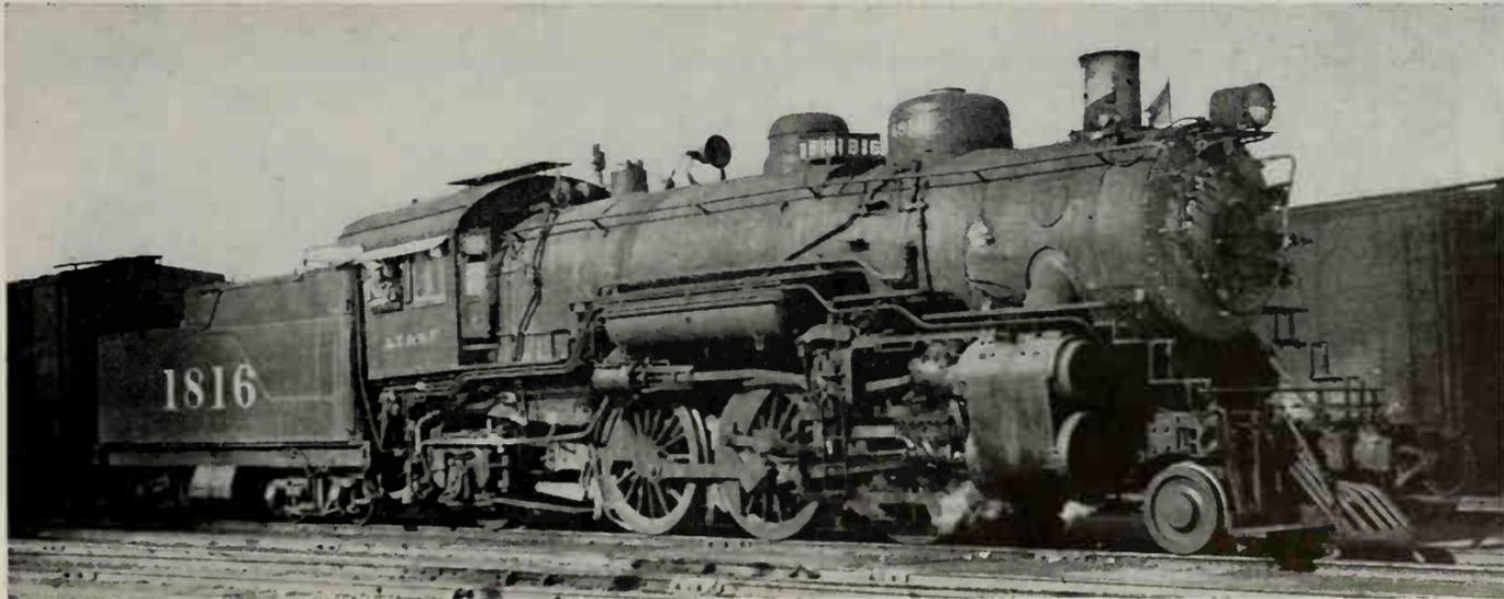
Atchison, Topeka & Santa Fe 2-6-2 (Prairie) Type Locomotive for freight service No. 1816. Built by The Baldwin Locomotive Works in 1906. Rebuilt by the A. T. & S. F. in 1928.
