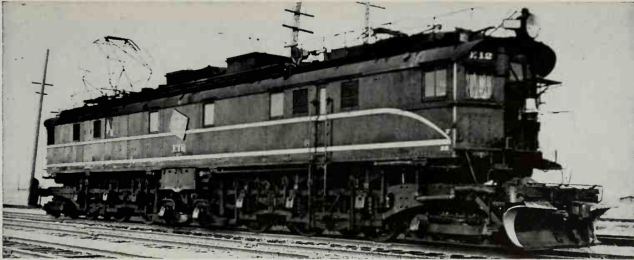
Chicago, Milwaukee, St. Paul & Pacific No. E-12, Class EP-3, 3,000-Volt D.C. Passenger Locomotive built by the Westinghouse Electric & Mfg. Co. and The Baldwin Locomotive Works in 1918. Nos. E-10 to E-19.
