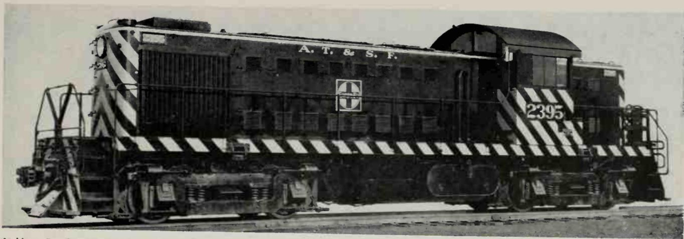
Atchison, Topeka & Santa Fe No. 2395; 1,000-Hp. Road Switching Locomotive built by American Locomotive Company-General Electric Company in November 1949.
