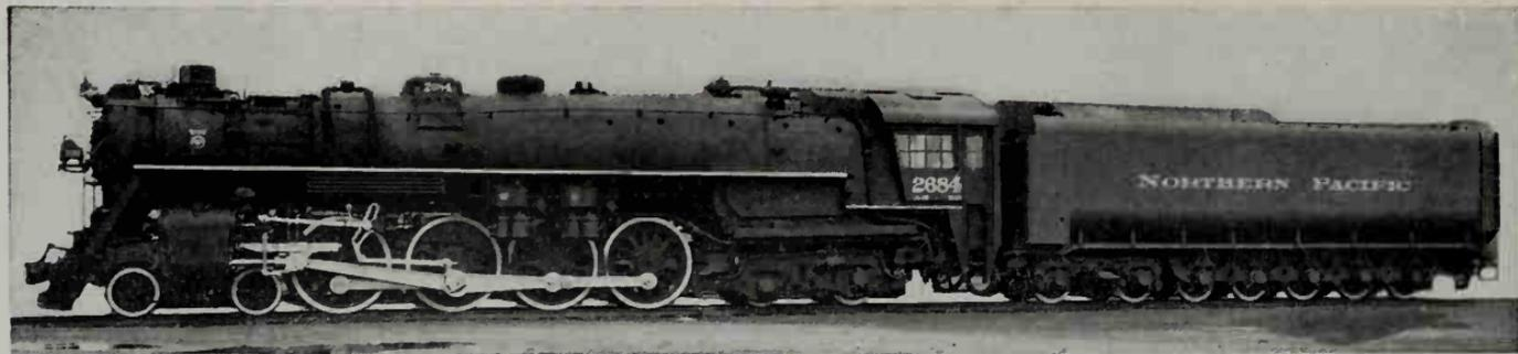
Northern Pacific 4-8-4 Type Locomotive for passenger service, Class A-5, Nos. 2680-2689. Built by The Baldwin Locomotive Works in 1943.
