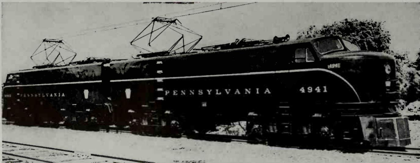
Pennsylvania No. 4941, Class E-2b, 111,000-Volt A.C., 2,500-hp. Freight Locomotive, built by the General Electric Co. in 1951.
