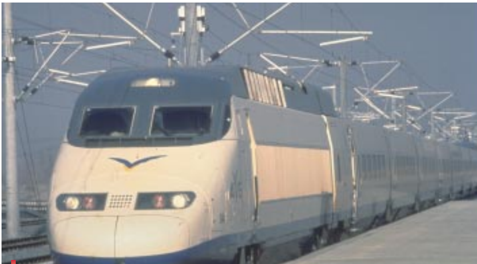
For Spanish infrastructure operator GIF, Alstom supplied power supply and catenary for AVE lines
