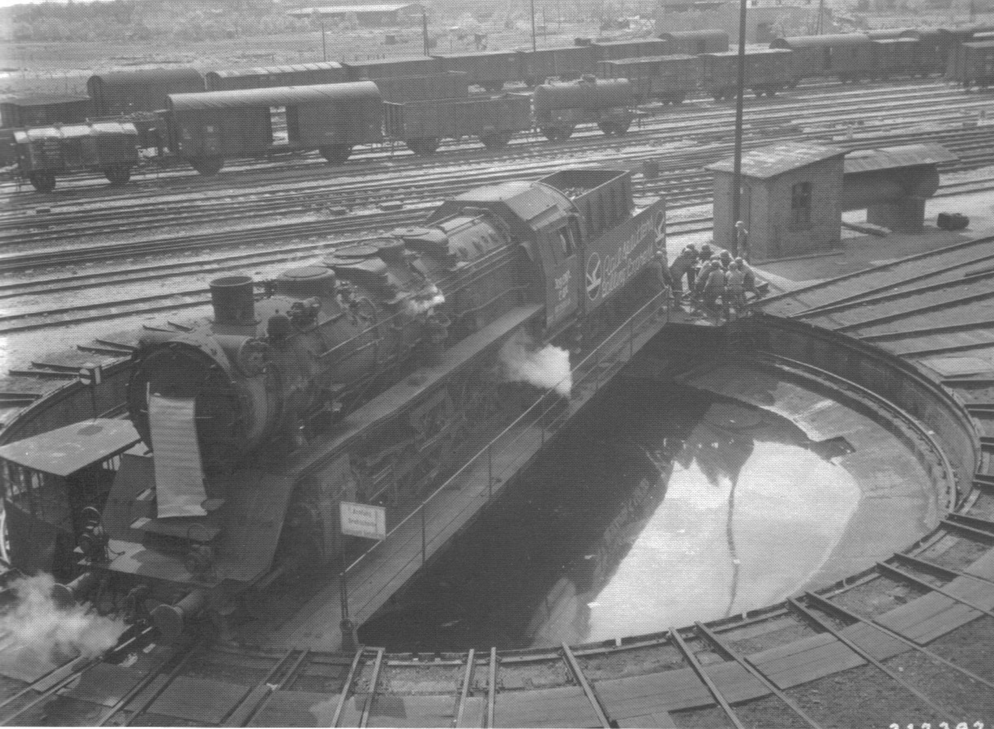
This turntable was manually operated by the 309th Combat Engineers, aided by displaced Polish citizens. The engine was used to convey supplies between Arendsco and Oebisfelde, Germany, for the 9th Army. (4-26-45)
