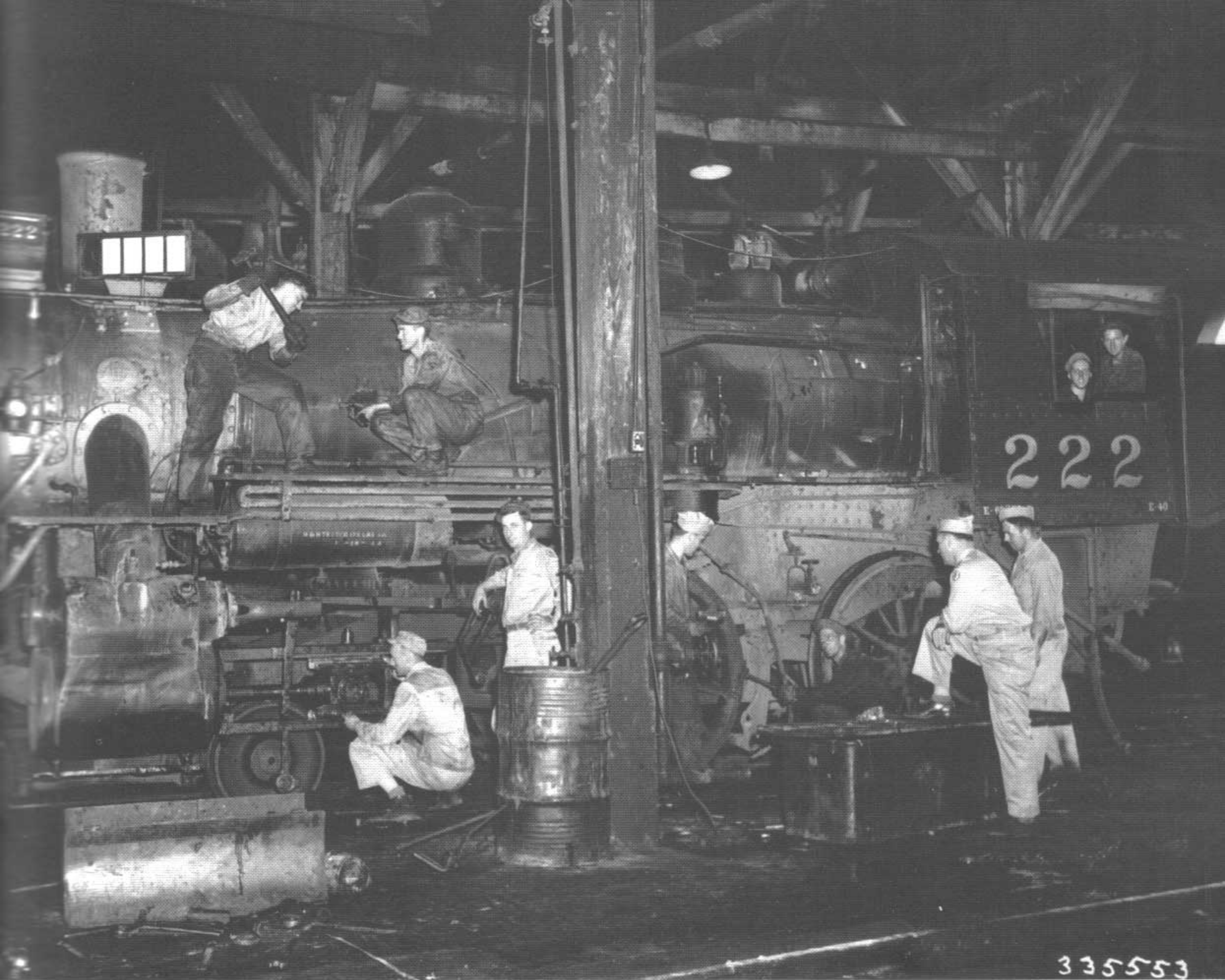
Members of the 716th Railway Operating Battalion put the finishing touches on an overhaul of engine 222 at Fort Sam Houston, TX. (5-11-44)
