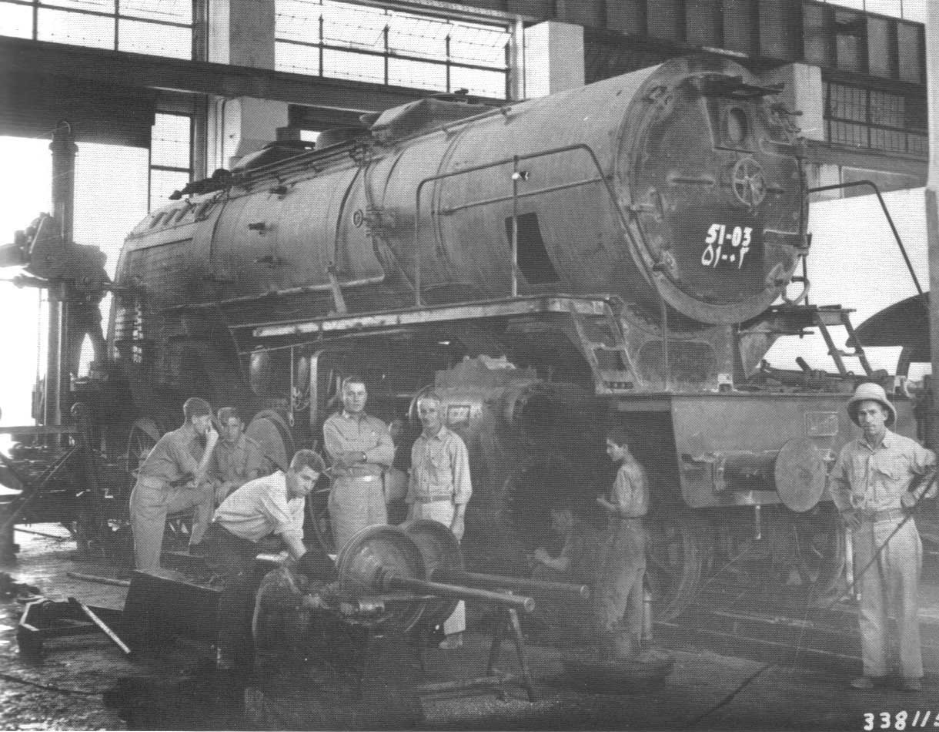
This locomotive was being repaired in the heavy machine shop of the Iranian State Railway. (9-30-45)
