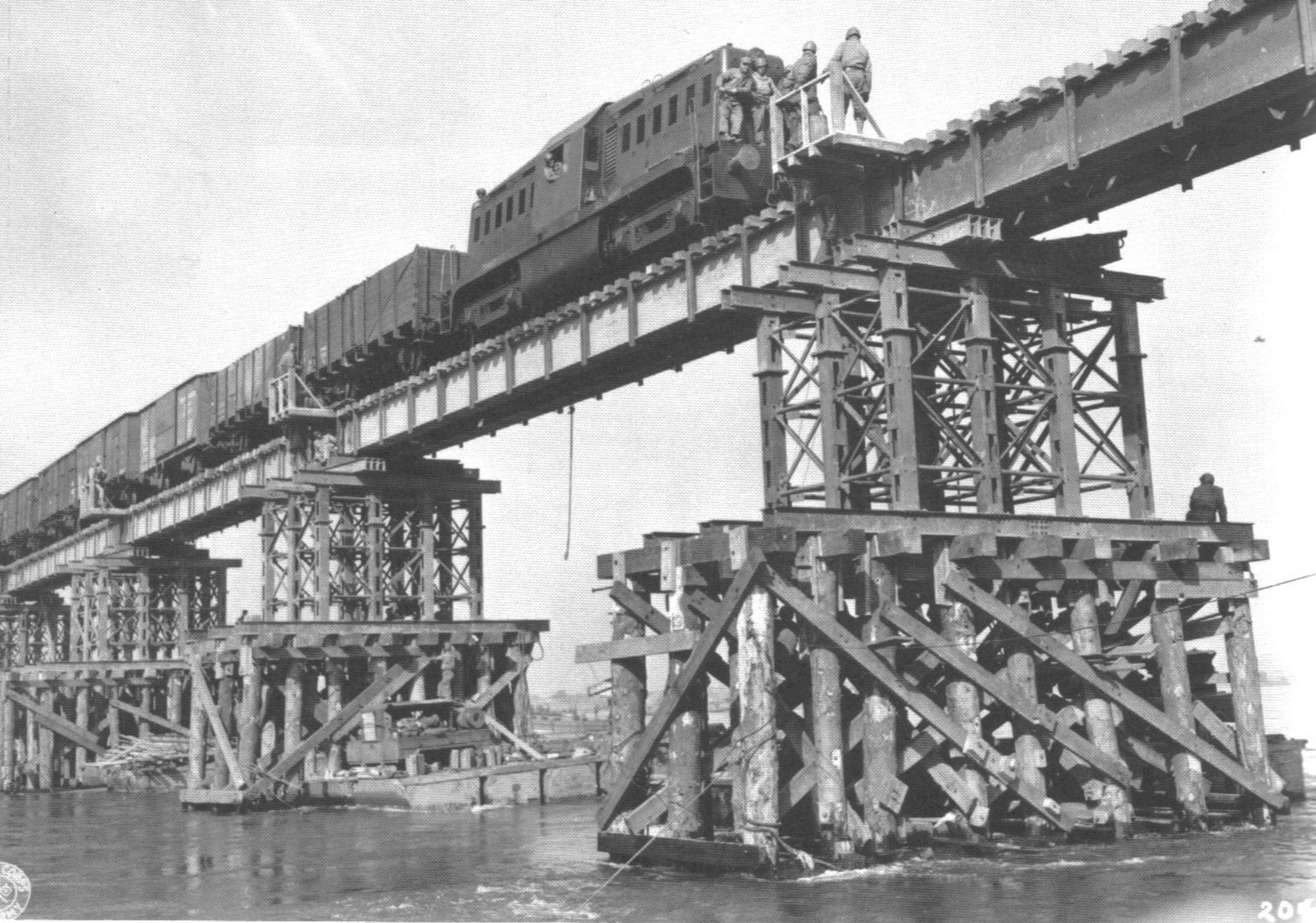
A Transportation Corps train moving across the Rhine at Wesel, Germany, on a bridge constructed by the U.S. 9th Army Engineers. (4-10-45)
