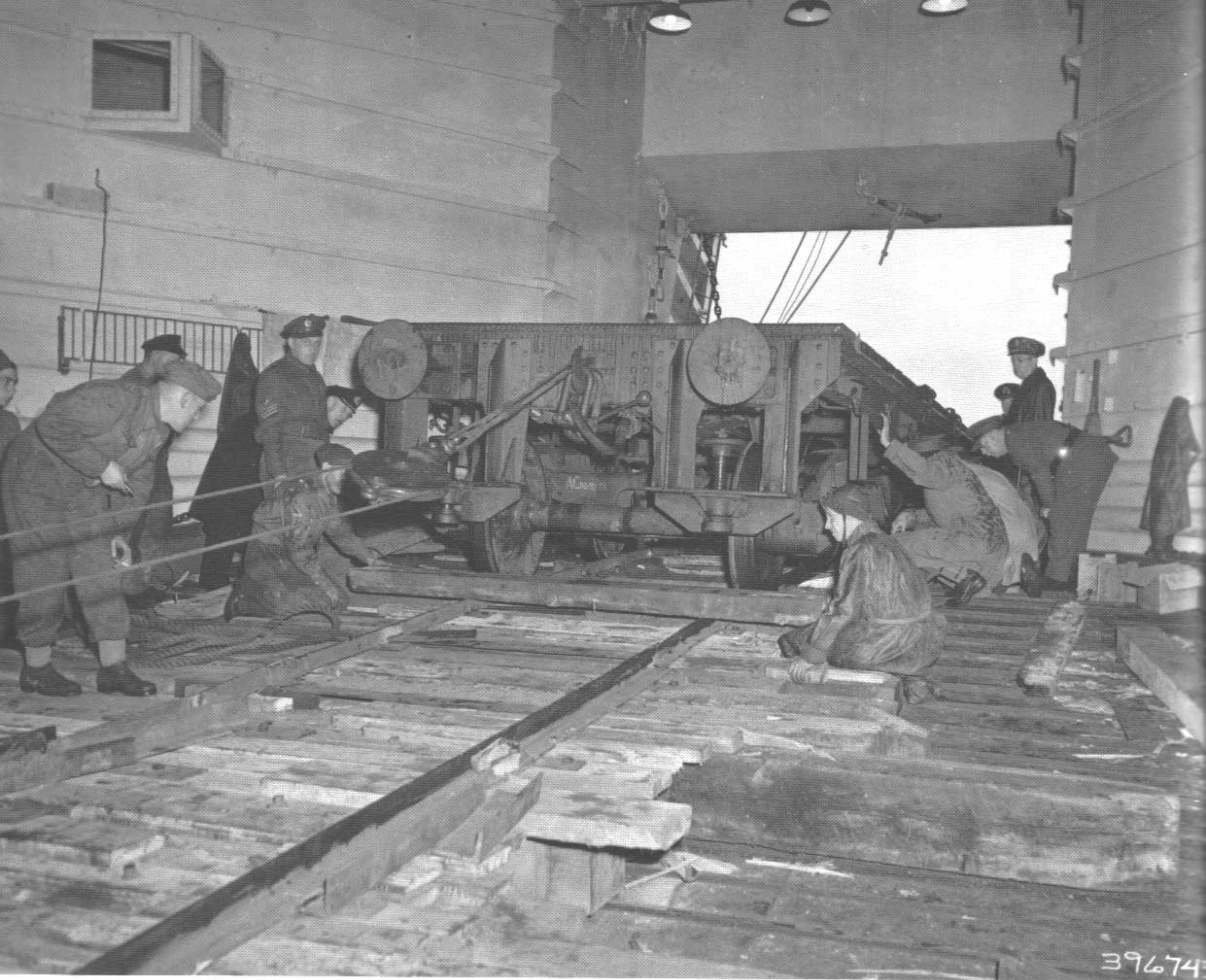
A successful experiment by Royal Engineers proved that tracks could be laid and rail stock loaded and transported aboard a tank landing craft. (9-7-43)
