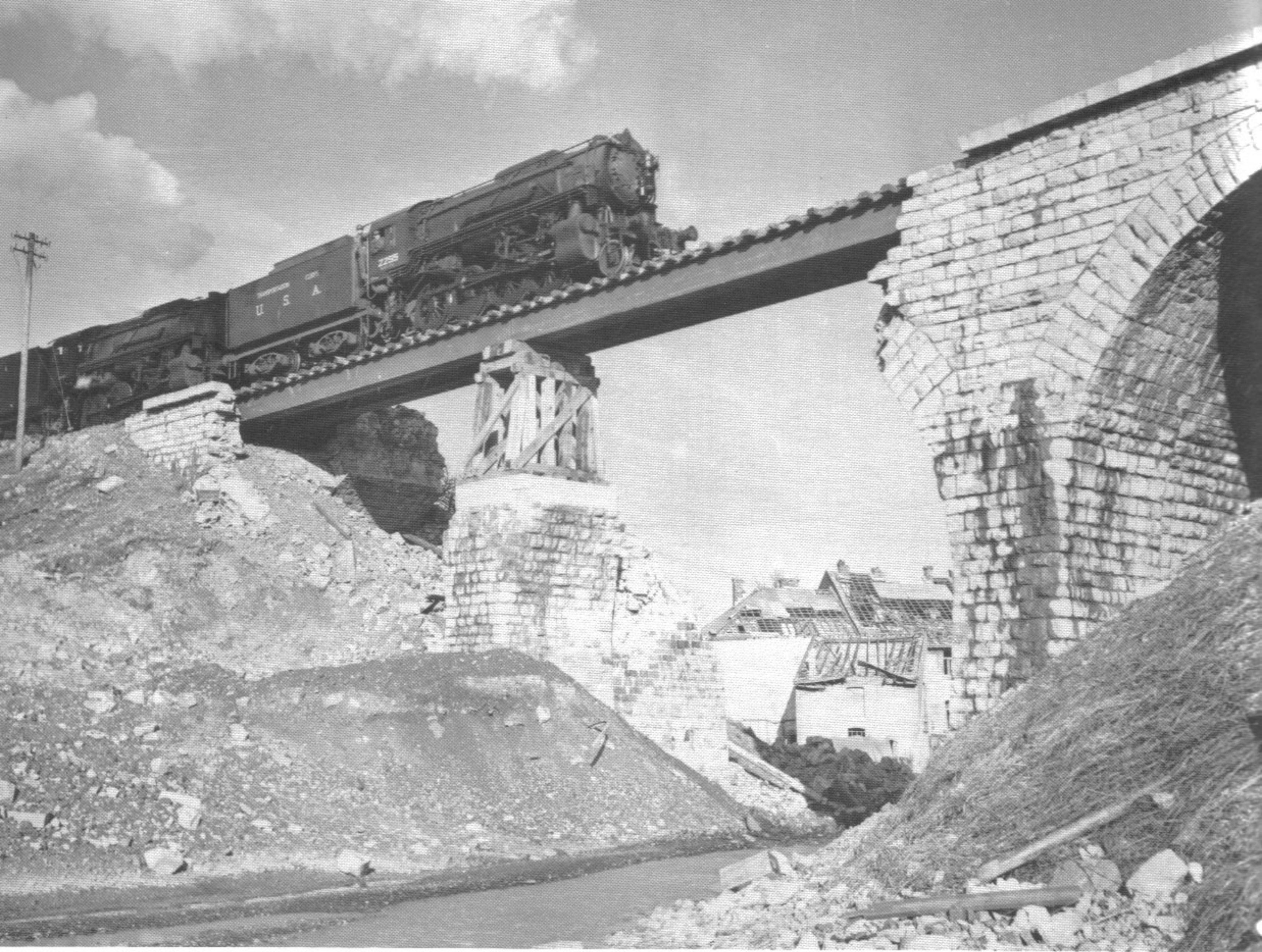
Two U.S. Army locomotives passing over a rebuilt viaduct to pick up a string of cars filled with gasoline, near Stolberg, Germany. (2-16-45)
