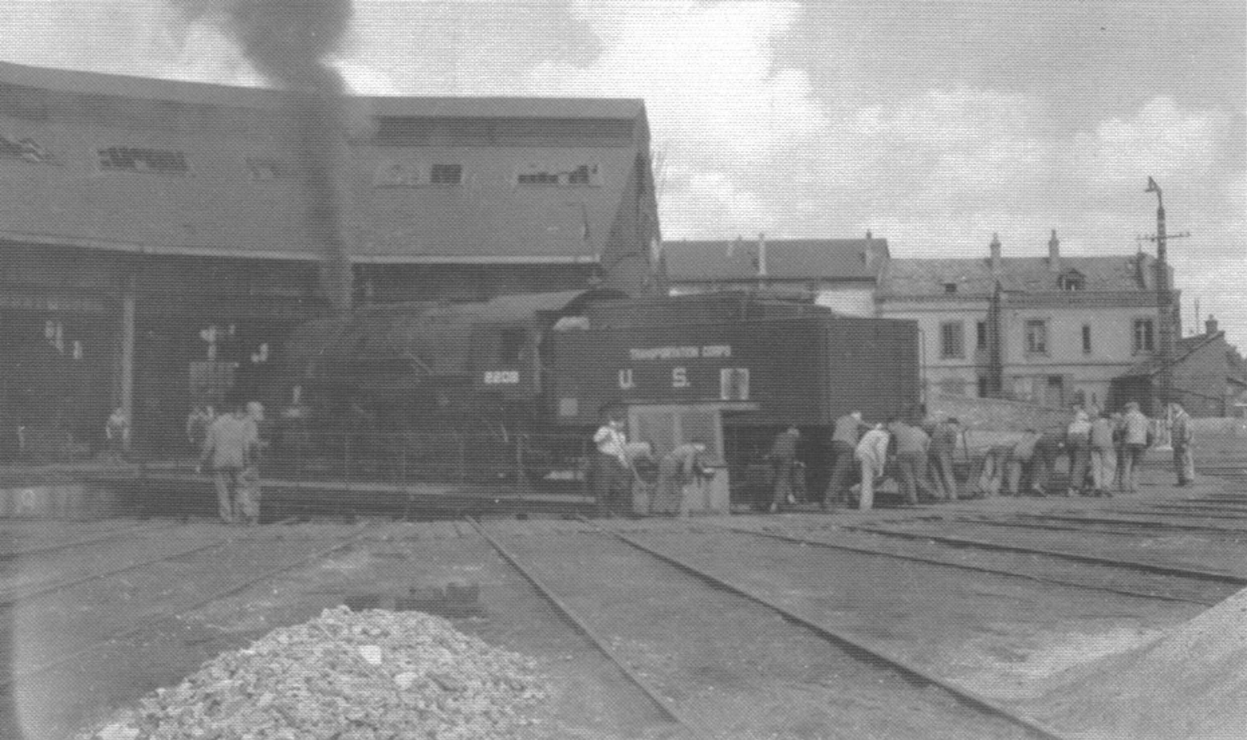
With no electric power available, French manpower was used to turn U.S. Army #2208 on the turntable at Chartres, France. (8-25-44)
