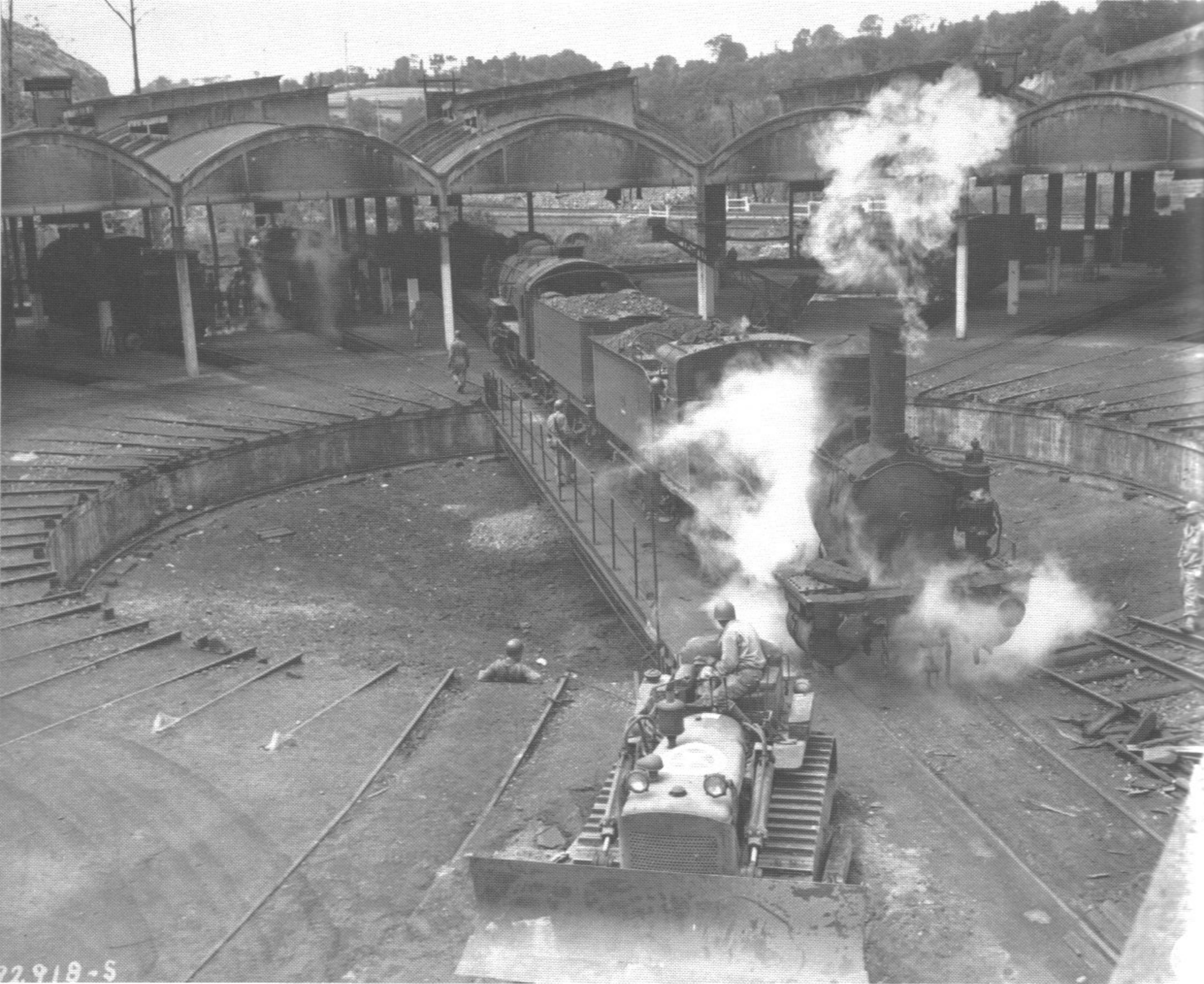
Without electric power the Americans use a bulldozer to move this French turntable. (7-15- 44)
