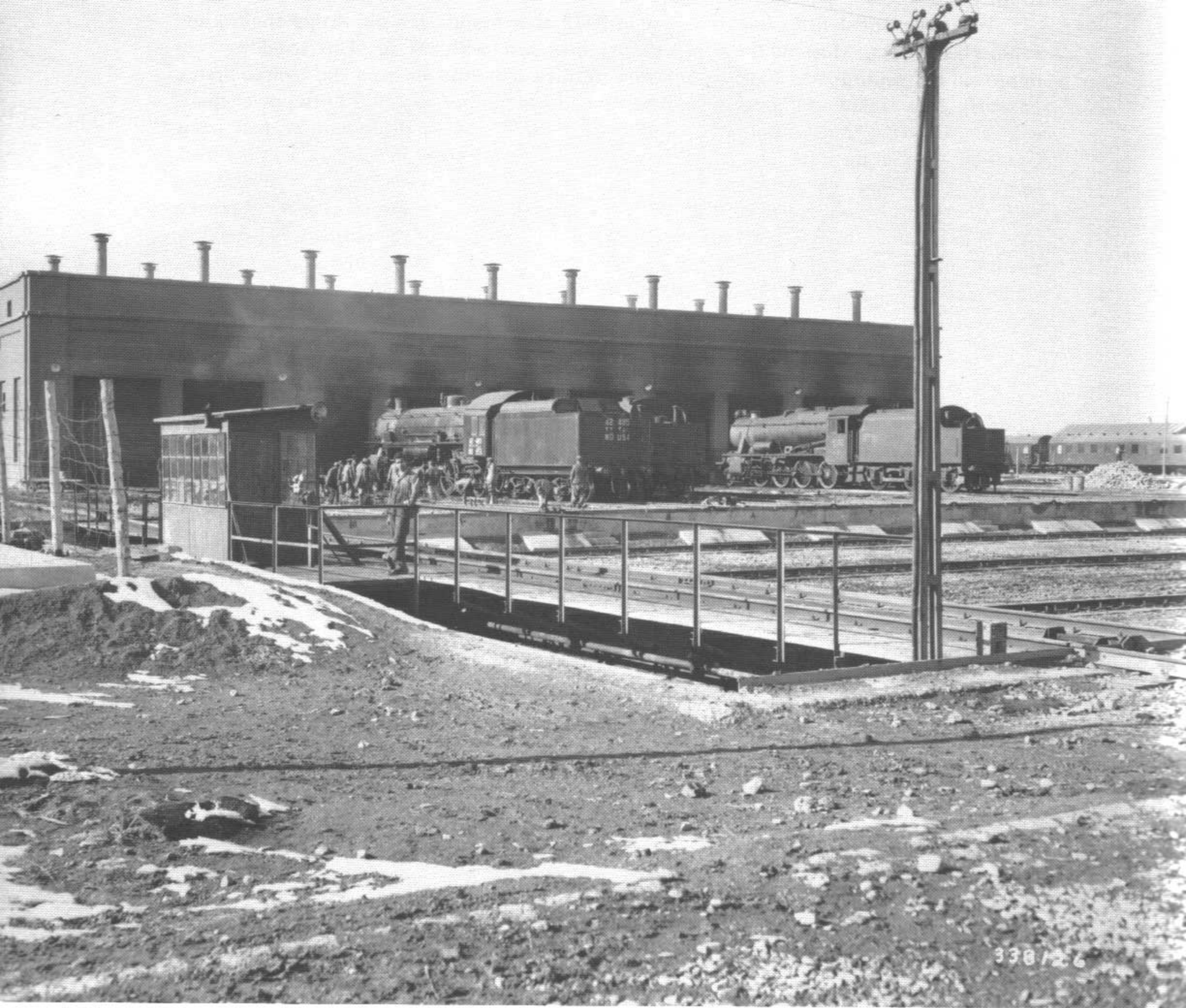
The transfer table behind the running shed at Camp Atterbury, Teheran, Iran. (1-8-45)
