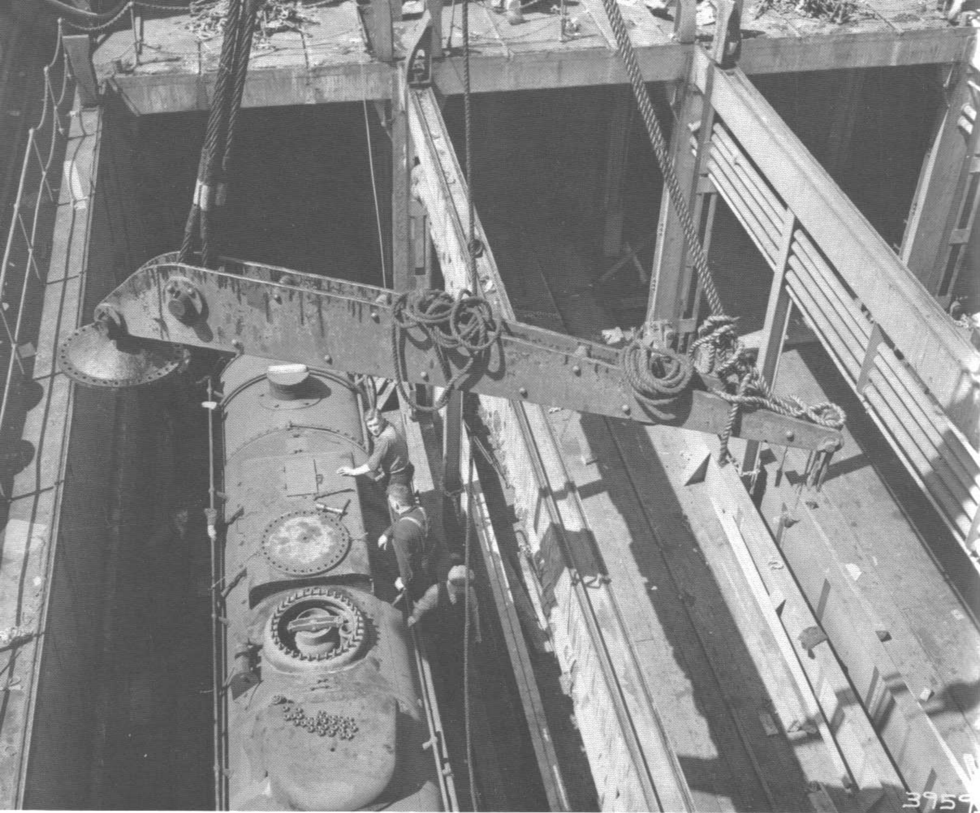
A lifting beam is lowered into position for attachment to a locomotive aboard the seatrain Texas at Birkenhead, England. (7-31-43)
