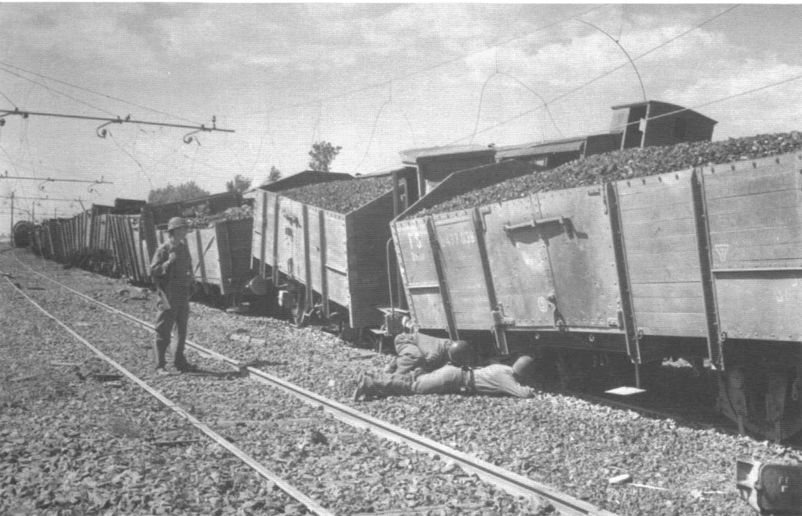
Blocked by the bombing of railroad bridges farther north, the Germans destroyed the trucks of these coal cars by placing demolitions in the journal boxes. (6-13-44)
