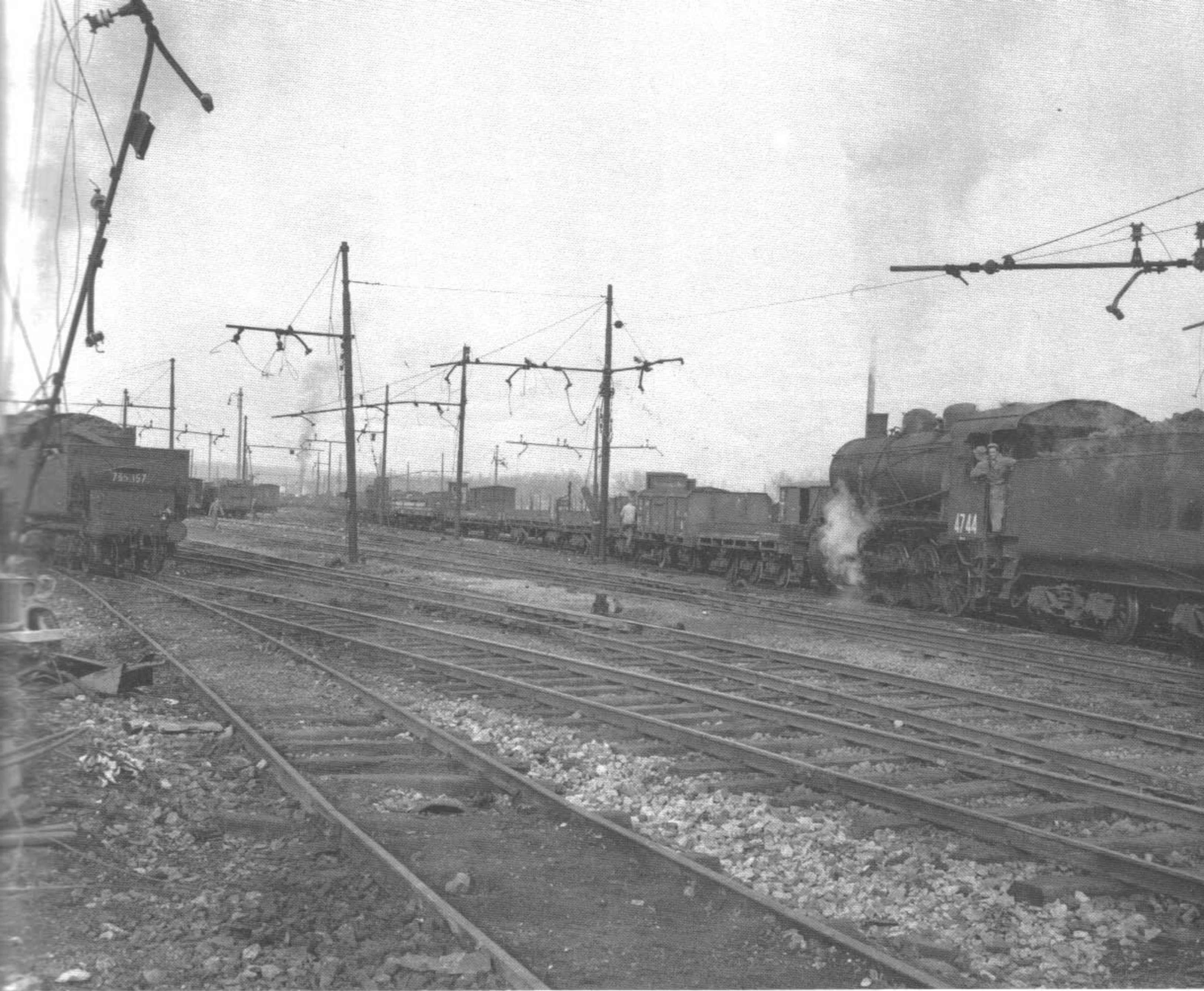
Train cars, reconstructed by the MRS, in the Naples railway yard. (12-11-43)
