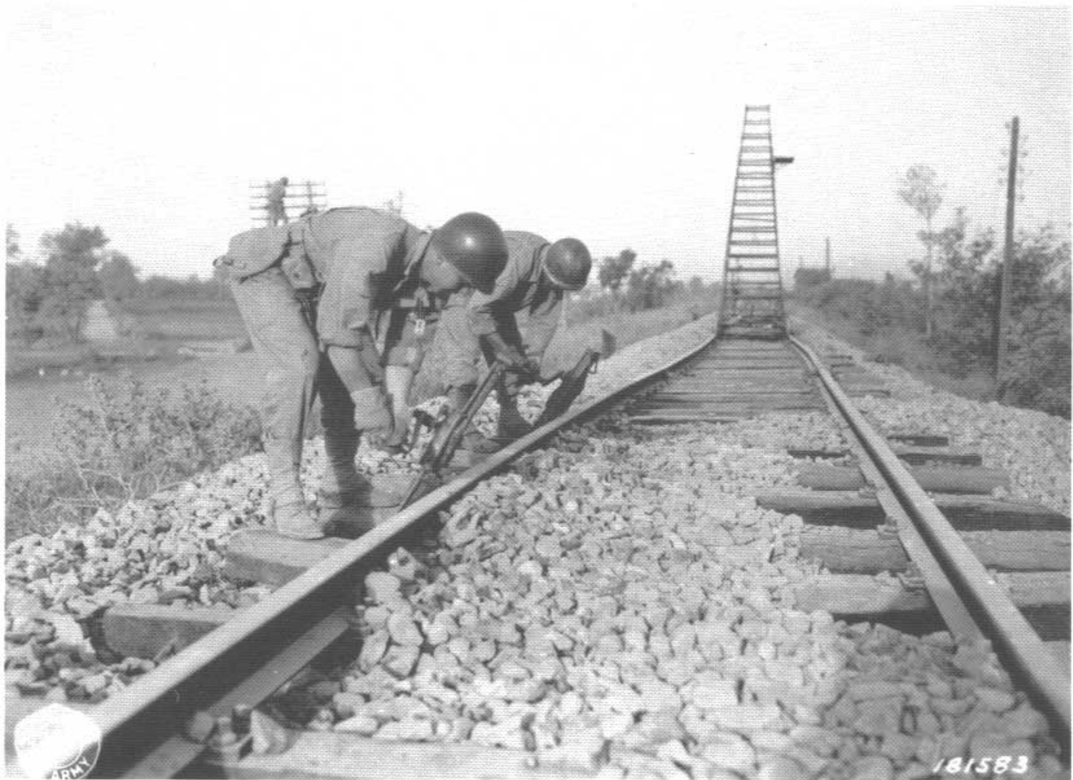
S/Sgt. M.E. Smith, Jakin, GA, and Sgt. Joe Wierzba, Bruce, WI, use jacks to straighten twisted rails near Battipaglia, Italy. (9-26-43)
