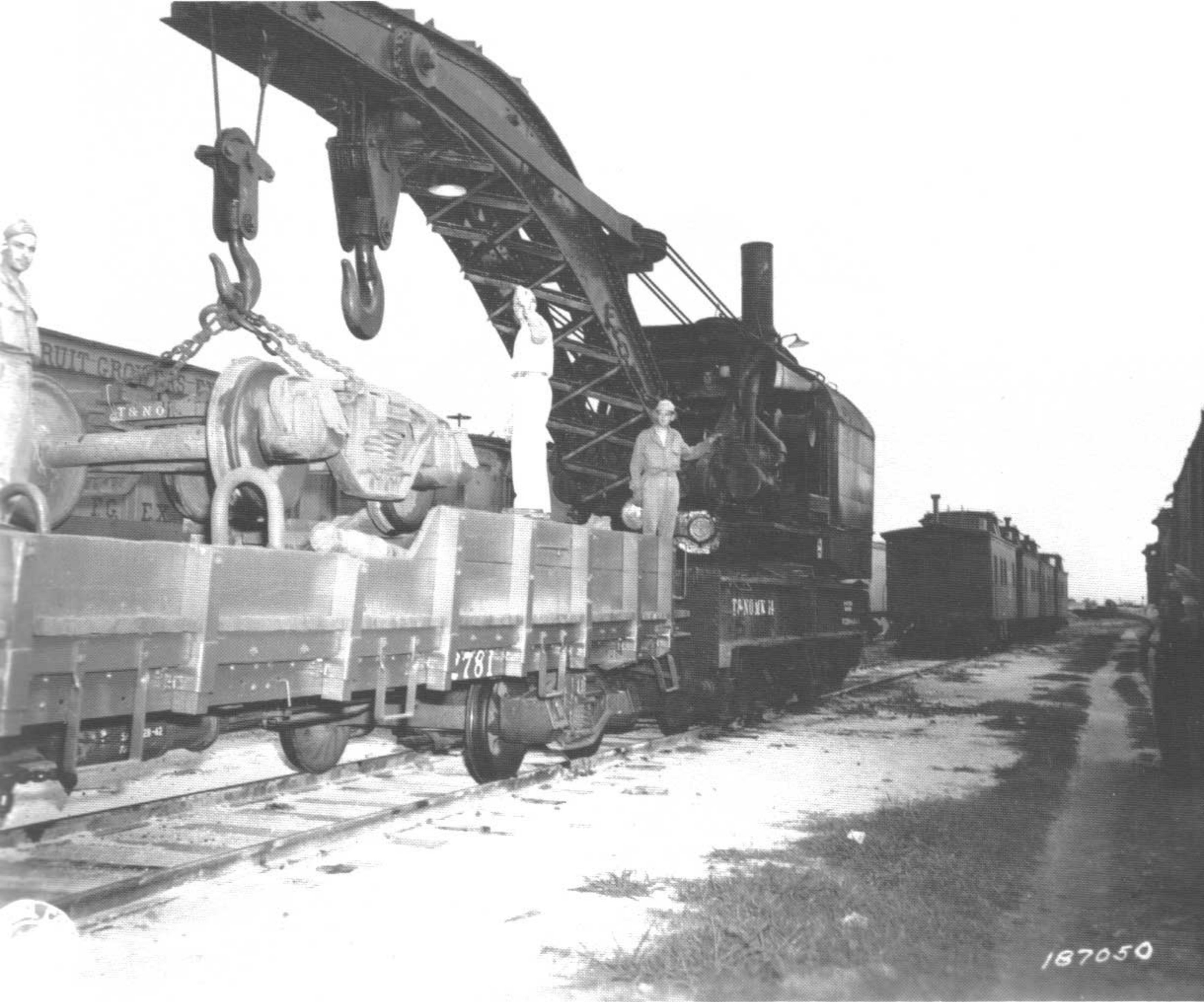
A railroad hoist crane is used to lift railroad wheels from a flat car at Ft. Sam Houston, TX. (7-9-43)
