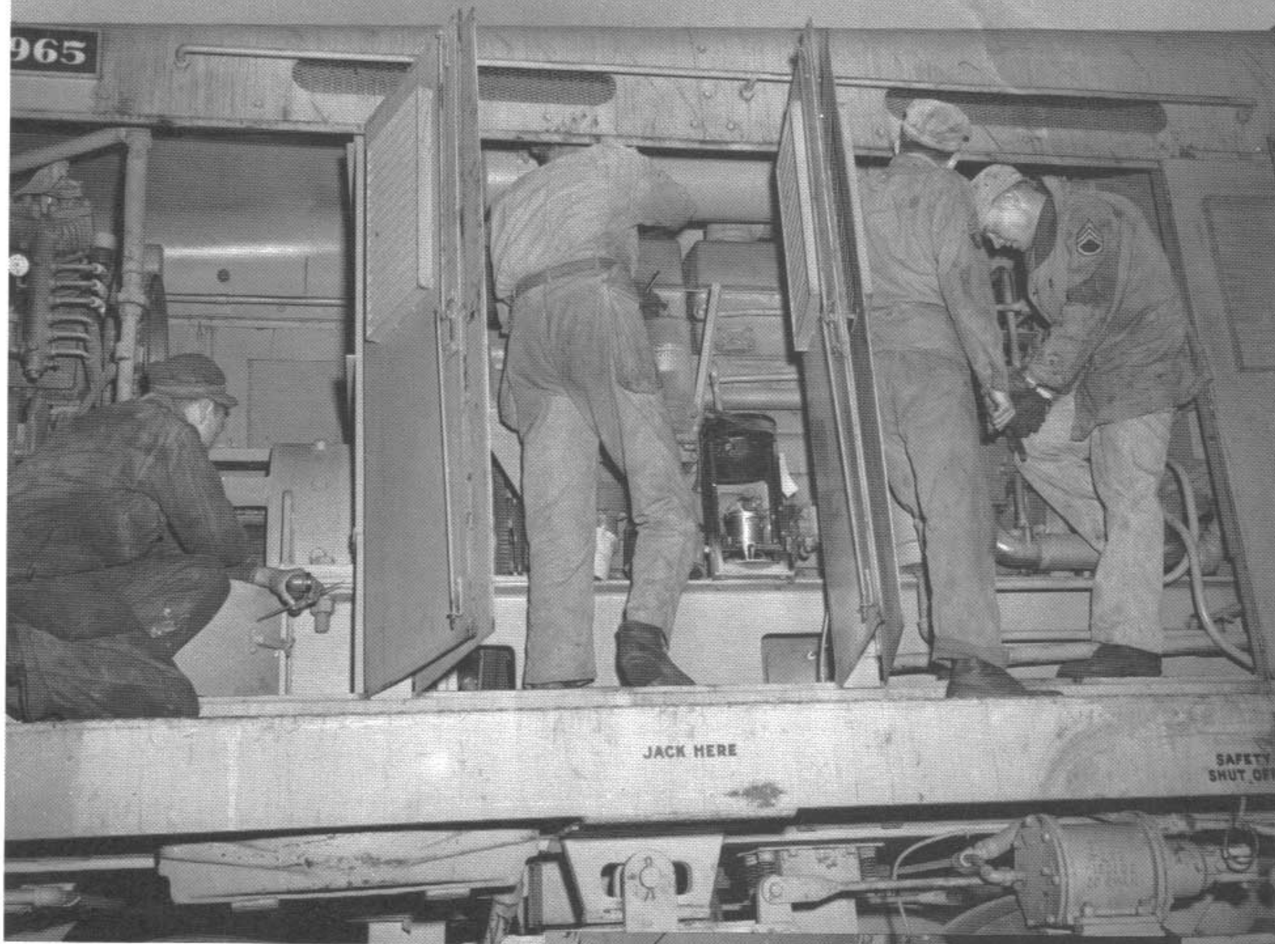
Enlisted men of the 751st Railway Shop Battalion reassemble a diesel engine after ship- ment to Britain. (2-10-44)
