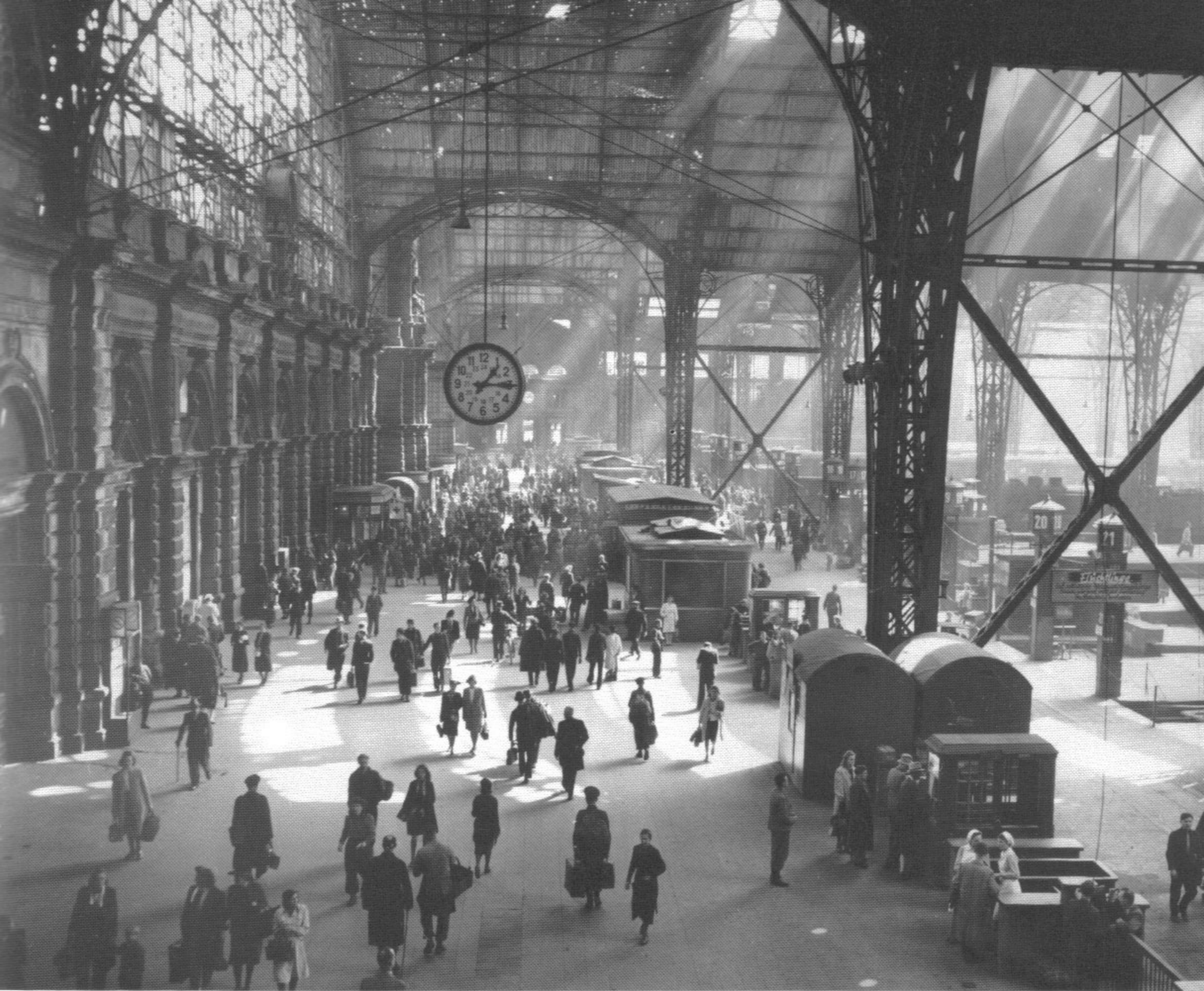
A view of one of the platforms inside the Main Station at Frankfurt, Germany, where despite repeated bombings, the roof structure survived, although not a single piece of glass remained. (4-4-46)
