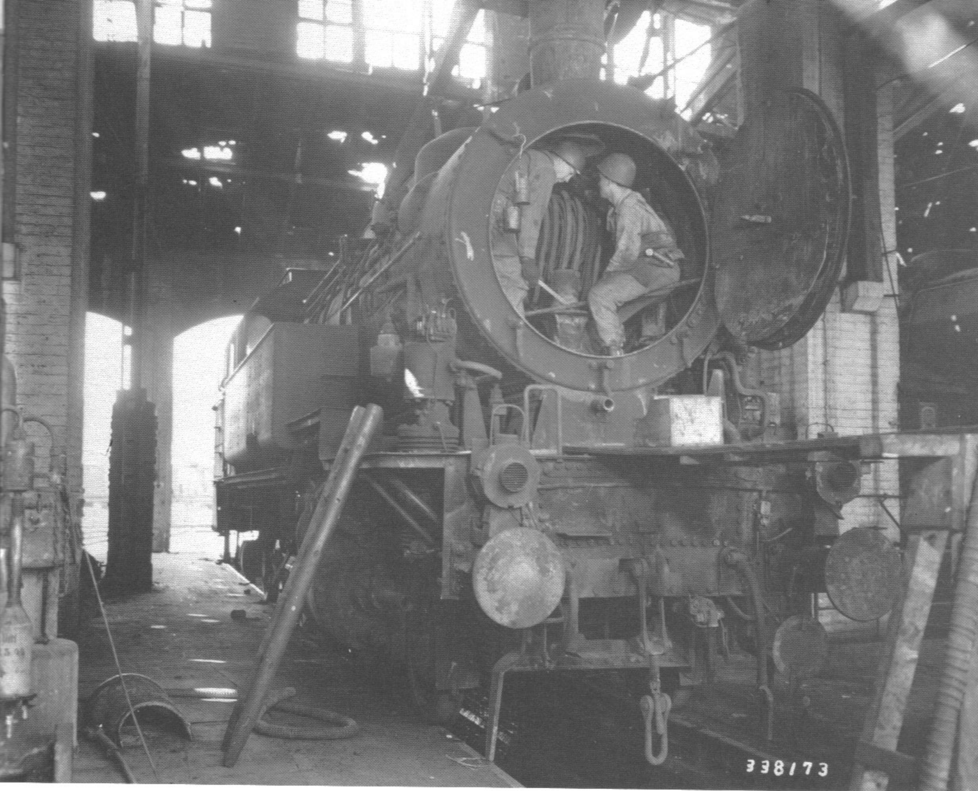
T/5 C.E. Fiske, Poplar Bluffs, MS, and T/5 A.H. Haines, Flat Woods, KY, working on one of 17 German locomotives repaired by the 746th Railway Operations Battalion within four days of taking over this roundhouse. (4-19-45)
