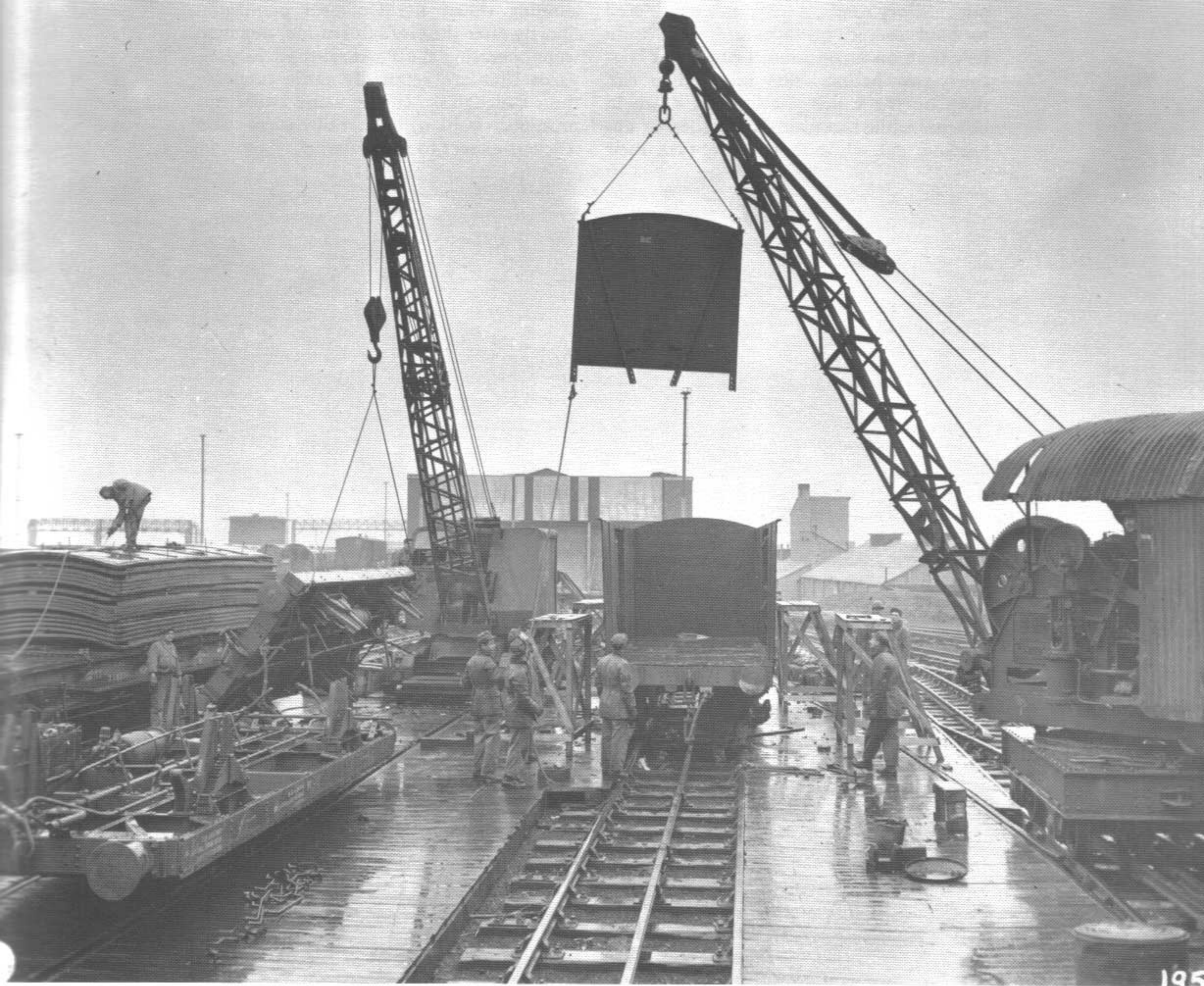
At an assembly line for the Transportation Corps rolling stock in England, the crane on the left inverts a completed under-structure while the crane on the right hoists a car end at the beginning of the car "out" line. (10-17-44)
